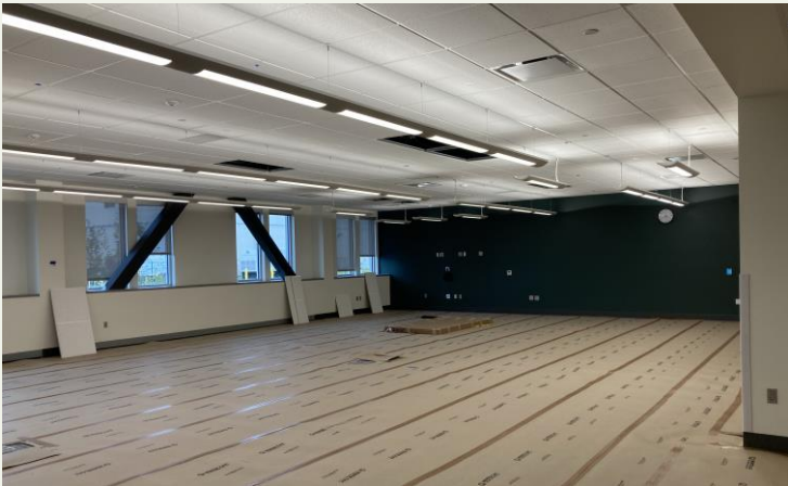
Open Office Area- (floor protection for furniture installation)
