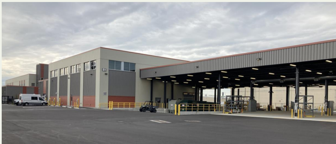
Loading Dock and Warehouse Facing West
