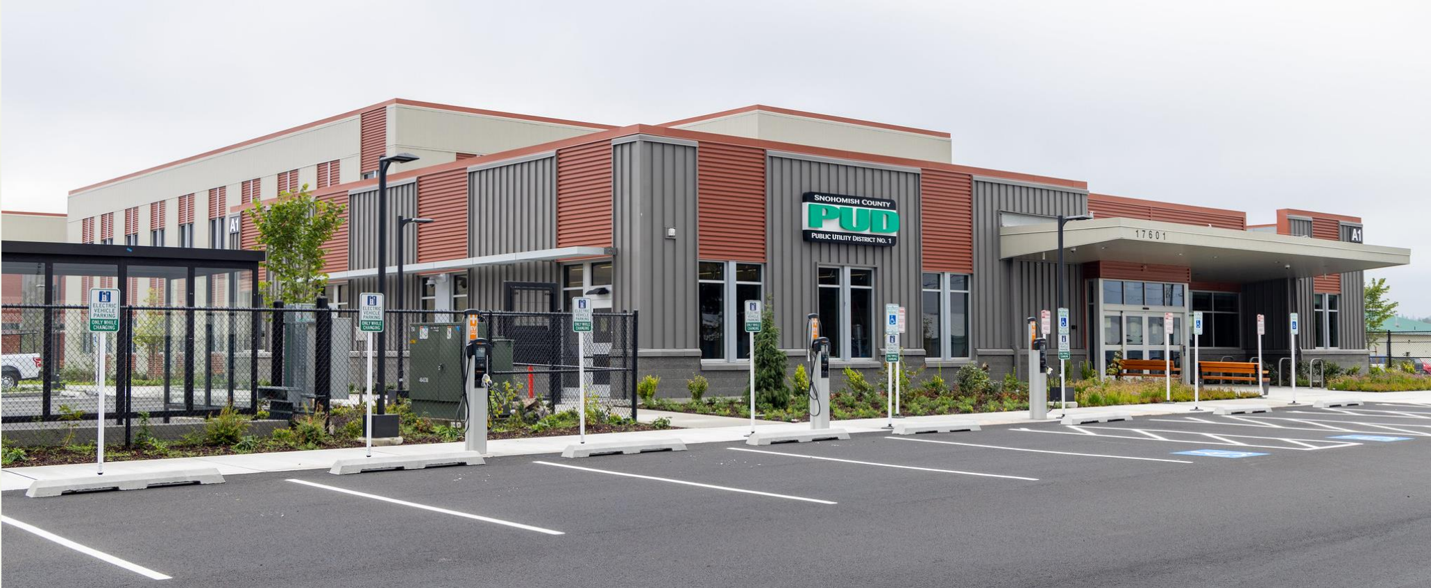
Office Facade (west face)
