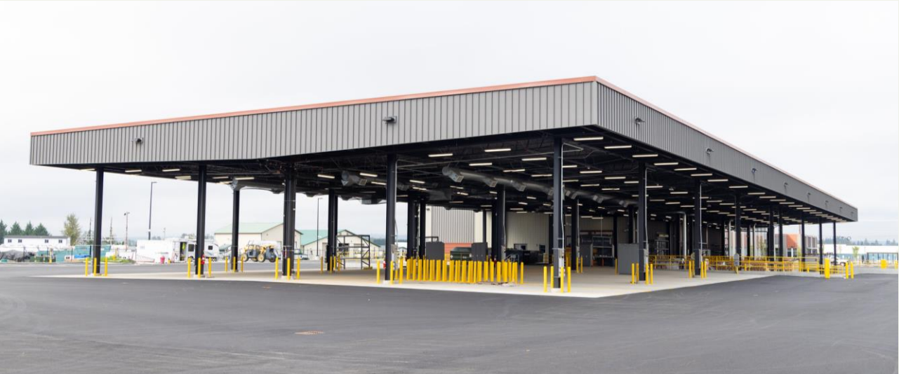
Loading Dock Looking West
