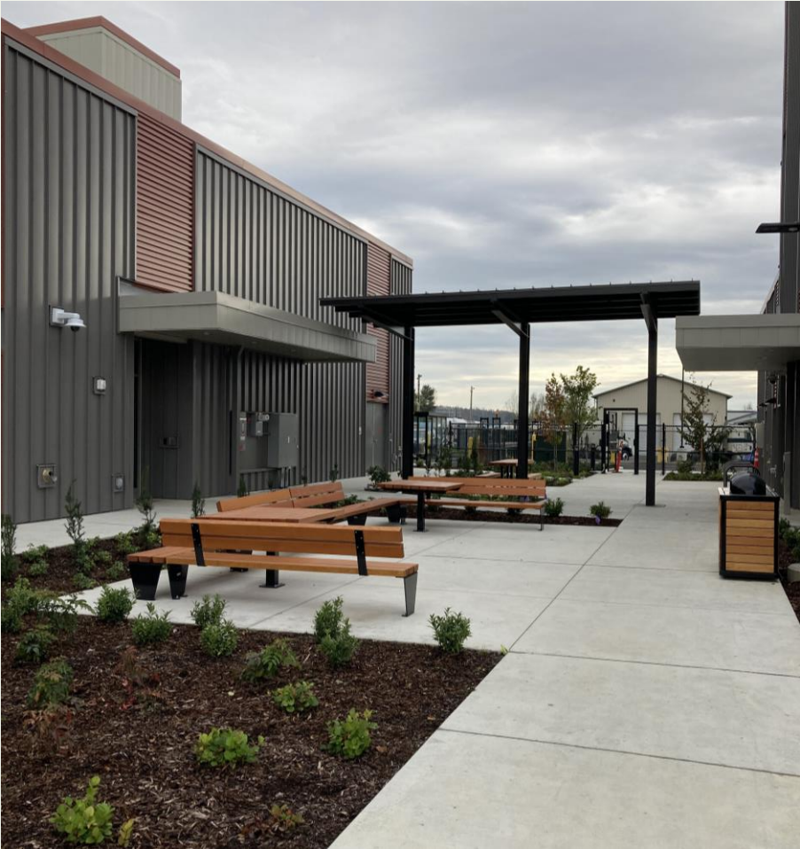
Breezeway Between Office and Warehouse
