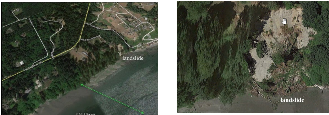
Figure 26. East shoreline of Whidbey Island showing Alt Route C and landslide
