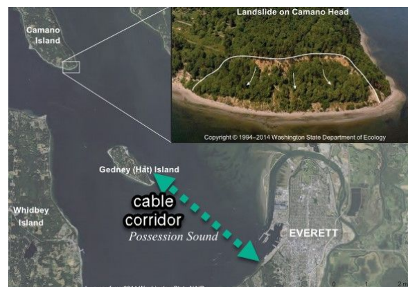
Figure 12. Landslide that inundated Hat Is.
